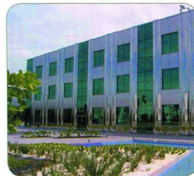
Grade 1.4521/444 brushed no. 4 (horizontal panels), Vivo Building, Rio de Janeiro, Nucleo Inox, Brazil (coastal environment)
