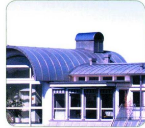
Grade 430Ti (standing seam technique), Ugine & Alz, Austria
